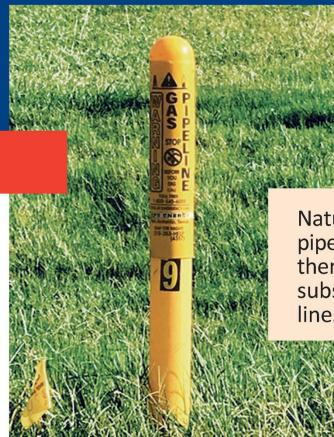
Natural gas pipeline markers are placed near pipelines, but not necessarily directly on top of them. Never use these markers or maps as a substitute for calling 811 to have all utility lines in your dig area located and marked.
