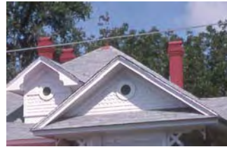
Soffits on Gable End and on Dormer
