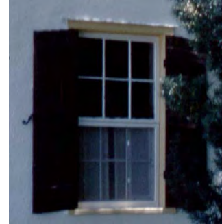
This six-over-six true divided light sash, double hung window is important to the period of the house. Also note that when closed the shutters cover the windows.
