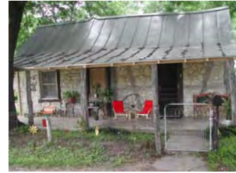
Wood frame and infill stone
