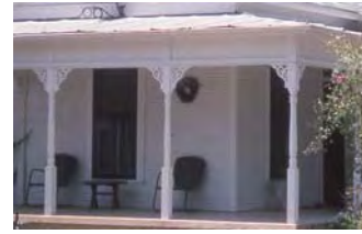
Columns with fan brackets
