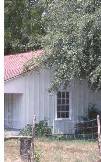
An example of board and batten siding.
