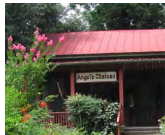
standing seam metal roofs of proper scale. The narrow width between the metal "seams," seen here is perfect for this small house.
