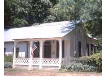
A porch built with the lateral addition to the older house, which is to the left.
