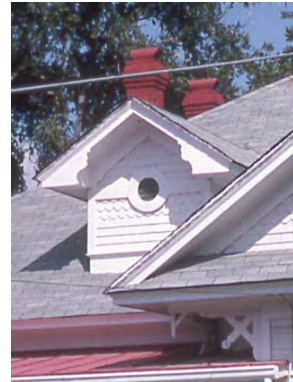
Boxed eaves, wheel window, and corbelled chimney caps
