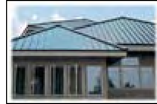
Not recommended: click lock metal roof panels because they're out-of-scale and dominate the roof ridge.
